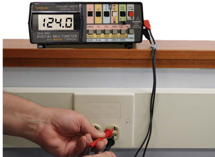
Outlet specifications: 120 VAC +/- 5% Range of 114-126 VAC
